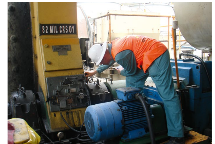
Vibration measurement at a ball mill drive
